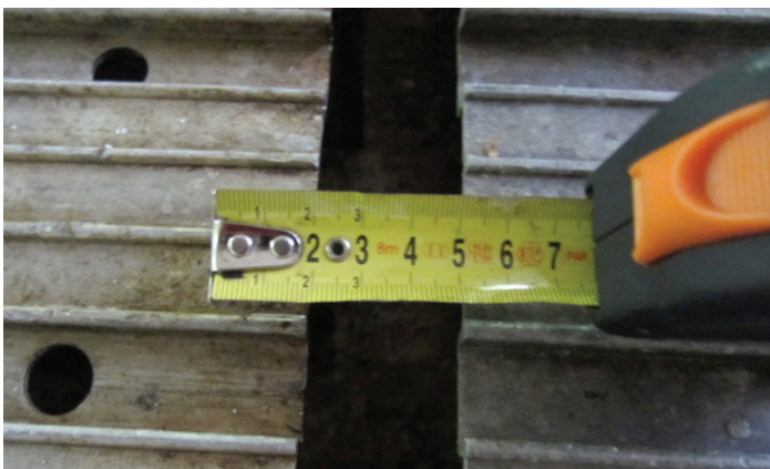
Measuring gaps in between aluminium gratings
